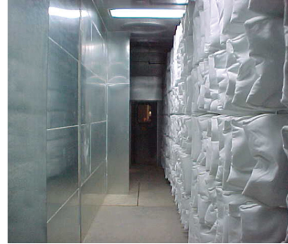
Paint Hangar Filter Bank
